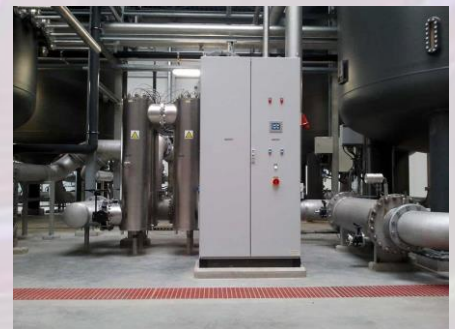
UV treatment for water preparation in Antwerp for Q_{\max.} 2 \times 500 \text{ m}^3/\text{h}
